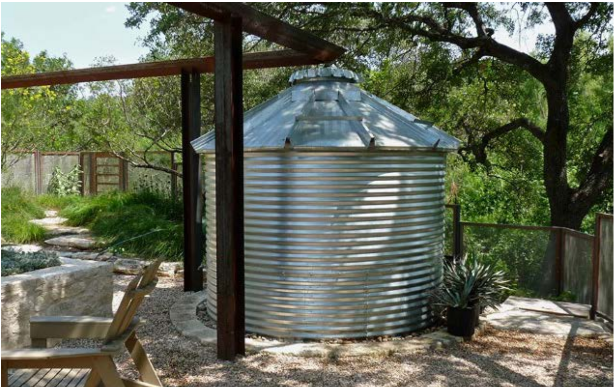
water tank in yard
